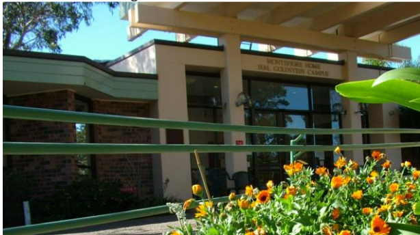
Picture 3 – Entry Foyer – External
